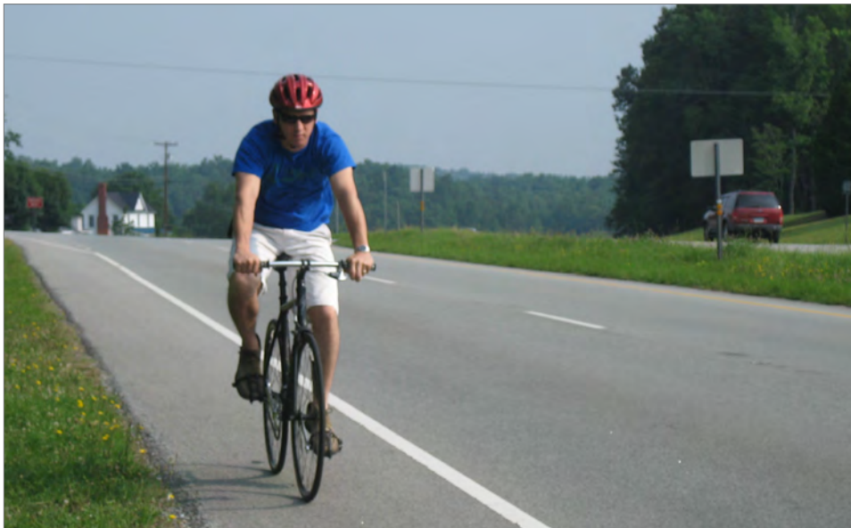
Paved Shoulder in Durham, NC. See Appendix A, page A-29 for paved shoulder design guidelines.
