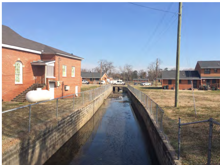
Portion of the “Ditch” with concrete channel through a public housing area at Elm Street.
