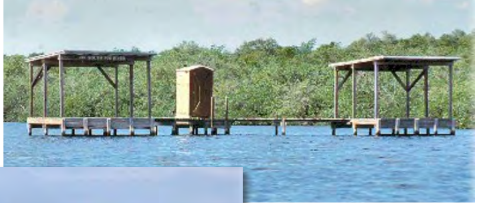
A Chickee Camp Site in Everglades National Park. Source: Seaside Water Trail Camping Platform Feasibility.
