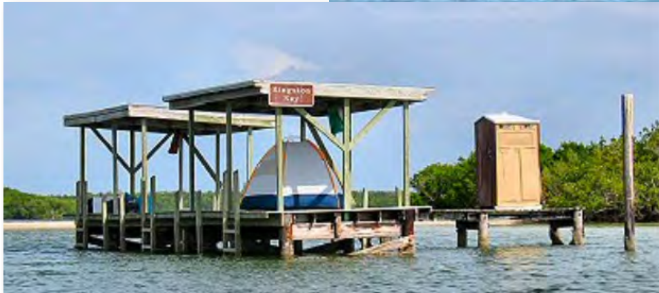
Docks with a shallow sloped roof supported by vertical posts with no wall structure. Source: Seaside Water Trail Camping Platform Feasibility.
