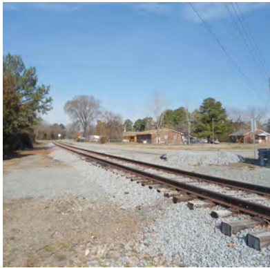
From left to right: US 117 at railroad crossing, railroad near Center Street at Elm Street, and George Street at railroad crossing
