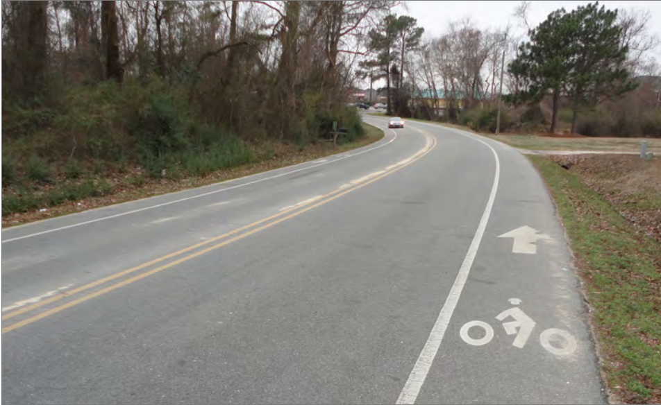
Bike lane on Harding Drive in Goldsboro. See Appendix A, page A-30 for bike lane design guidelines.
