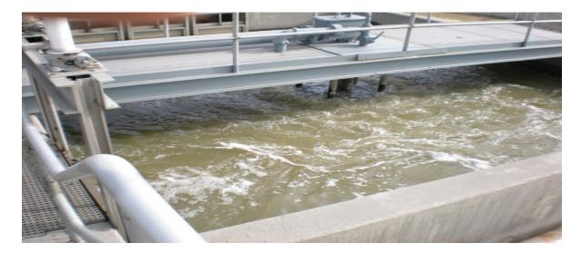
A diffused air system is utilized for transferring oxygen to the wastewater. Networks of membrane diffusers are installed within the main aeration channel. When air is diffused through the network, millions of tiny air bubbles rise to the surface and transfer oxygen to the contents of the tank.
