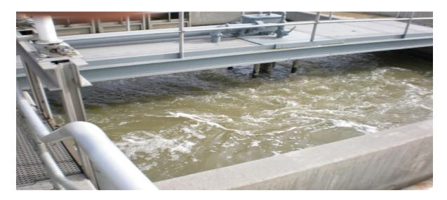
A diffused air system is utilized for transferring oxygen to the wastewater. Networks of membrane diffusers are installed within the main aeration channel. When air is diffused through the network, millions of tiny air bubbles rise to the surface and transfer oxygen to the contents of the tank.
