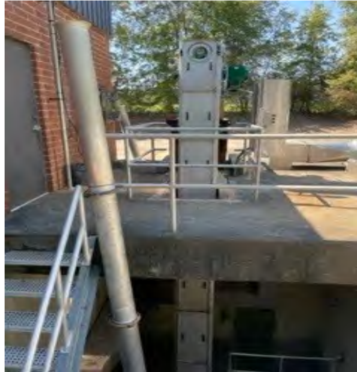
New Hope L/S Bar Screen Replacement $335,400 Completed.
