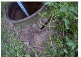
Manhole w/active infiltration (stains)
