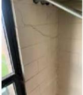
Exterior south wall of PD/Fire gym additional crack.
