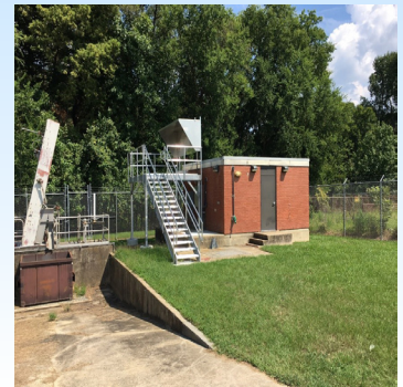
New raised platforms for electrical controls.
