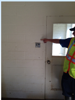
High water mark inside pump station.
