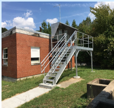
New raised platforms for electrical controls.
